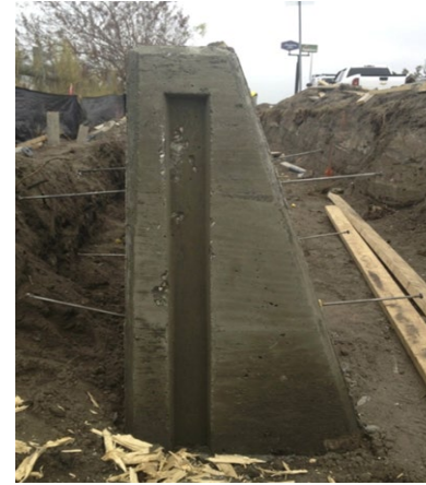
Gravity Retaining Wall
