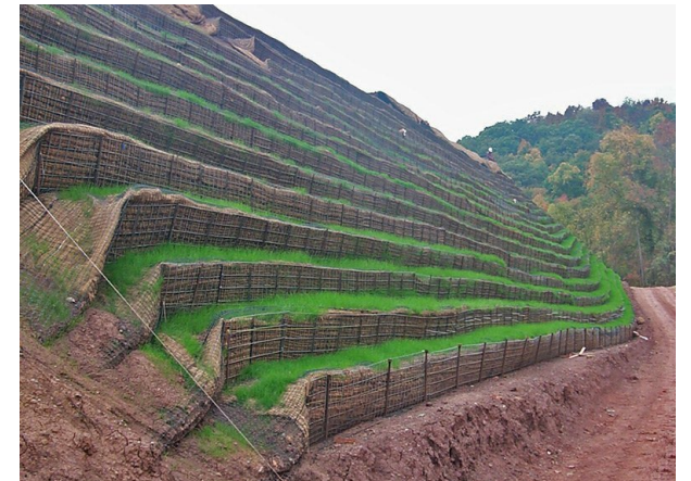
Reinforced Soil Slopes
